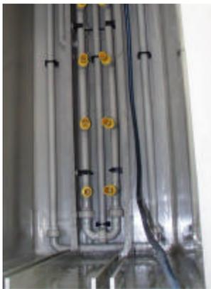
**Figure 5 - Installation of Educators in a Plating Cell**
