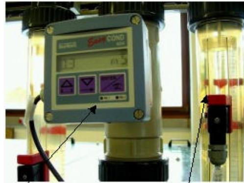
**Figure 19 - Conductivity Control/Flow Meter with min/max Alarm**
