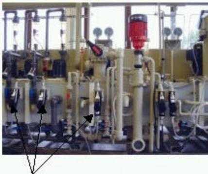
**Figure 18 – Pumps Which Can Be Plugged for Quick and Easy Replacement**
