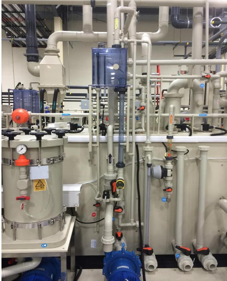
**Figure 22 – Etch Recycling System**
